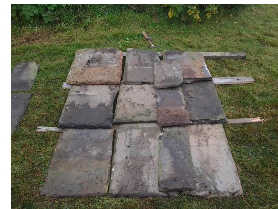
Reconstruction flagstone roof showing seamer method
